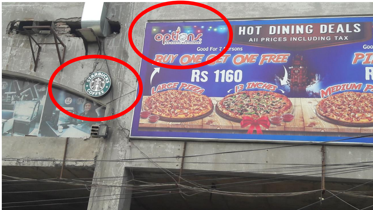
Photo. No. 01 – View of the Undertaking’s Restaurant from Outside the Building
