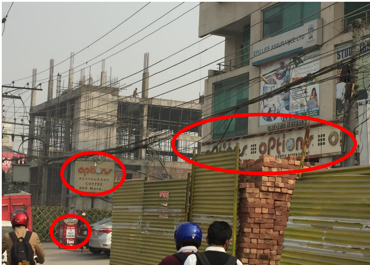
Photo. No. 01 – View of the Undertaking's Restaurant from Outside the Building
